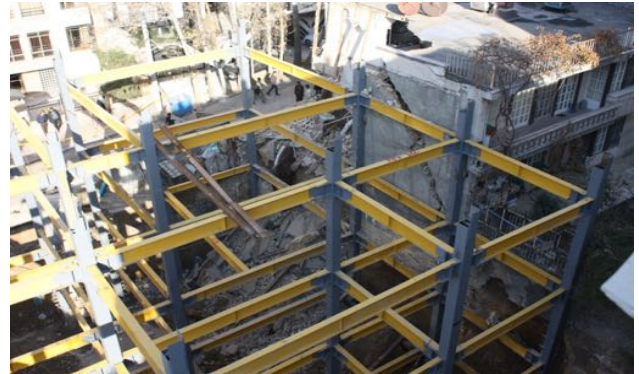
IOM Building Earthquake Resistance Assessment
